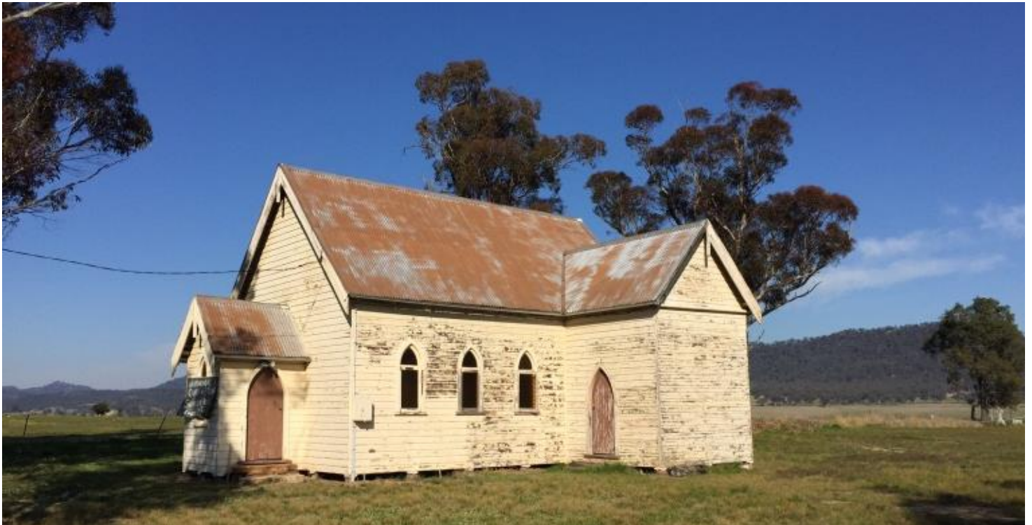
Former Upper Bylong Catholic Church
