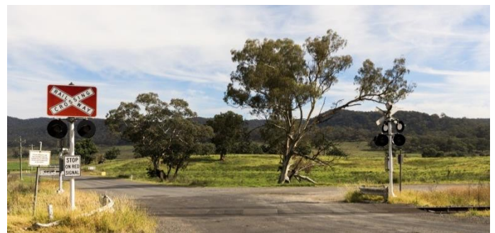
Typical railway crossing
